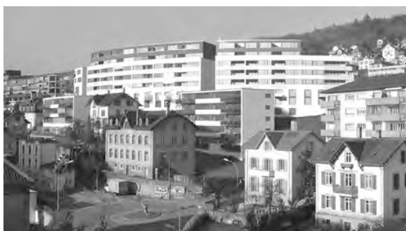
Figure 4: View of the apartment buildings on the East part of the site (doc. Bauart).
