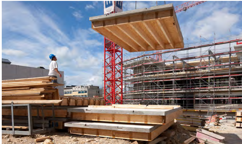
Figure 4. Assembly of the hybrid elements on site (Picture: Yves André).
