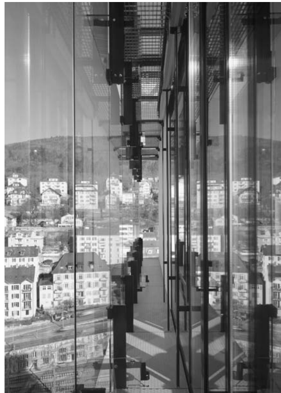
Figures 5-6 : Detail section of the double-skin façade (document Bauart) and view of the interstitial space (photo Th. Jantscher)
